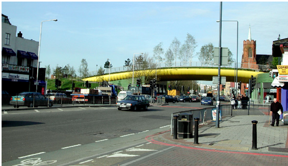
The Green Bridge
